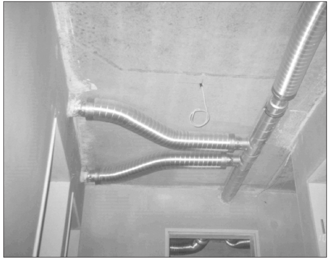
Figure 4.2.4 (Left) Optimized ground plan of an apartment in a social house project in Kassel, Germany; (right) a view of the air ducts
