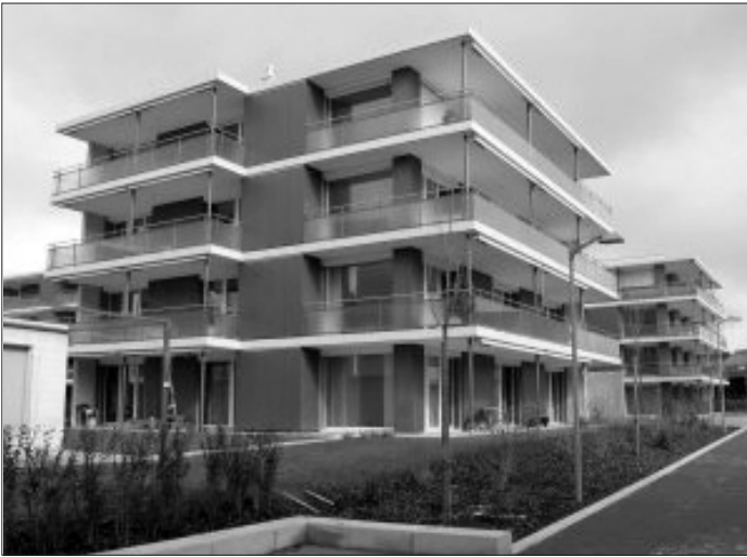
Figure 6.3.4 A passive house block as it was constructed
